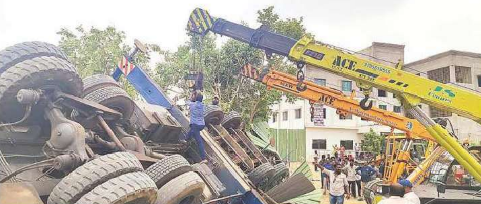
Efforts are underway to remove the crane from the pit in Tirupati on Tuesday
